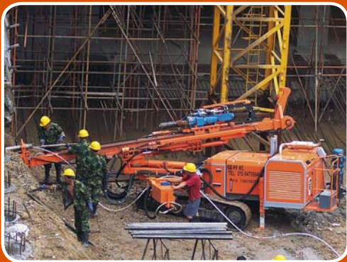
China - Anchor Drilling \phi 152.0\text{mm} China - Ankerbohren \phi 152.0\text{mm}
